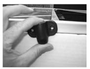
sure that the open socket portion of the bracket is flush to the top of the railing. Mark screw locations with pen or marker; Drill mounting holes with 5/32" bit. Secure bracket using two #10 x 3/4" screws and Phillips screwdriver. Measure along that same railing, 28" from the center of the first bracket, to locate the second mounting bracket. Position that bracket and secure to the rail with screws as above. Repeat for a third mounting bracket - again located 28" on center from the second.
